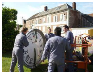
Installation Eglise Laversines (60)
